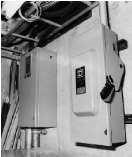
A new safety switch (right) will soon replace the old conductor box on the left. Conduit (metal tube) leads down to the safety switch; the conductor box lacks conduit. The safety switch can be locked out, while the box has no place for a lock.
