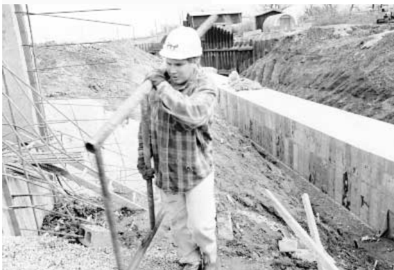
Workers remove forms from the tunnel's construction site.
