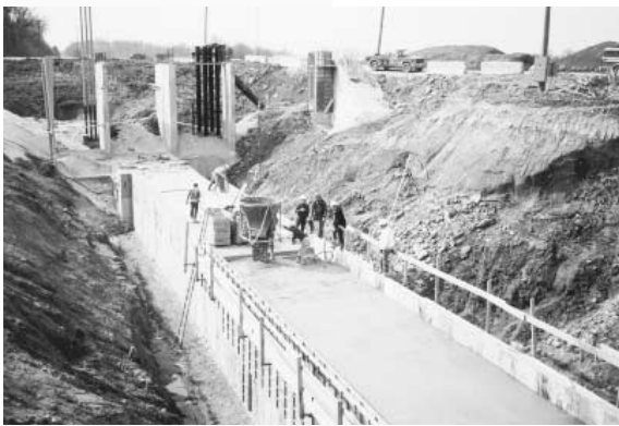
Workers remove forms from the tunnel's construction site.
