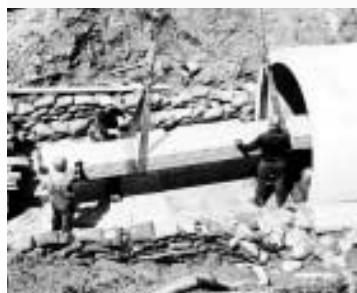
The first magnet of the Main Ring is lowered into place, April 1970.
