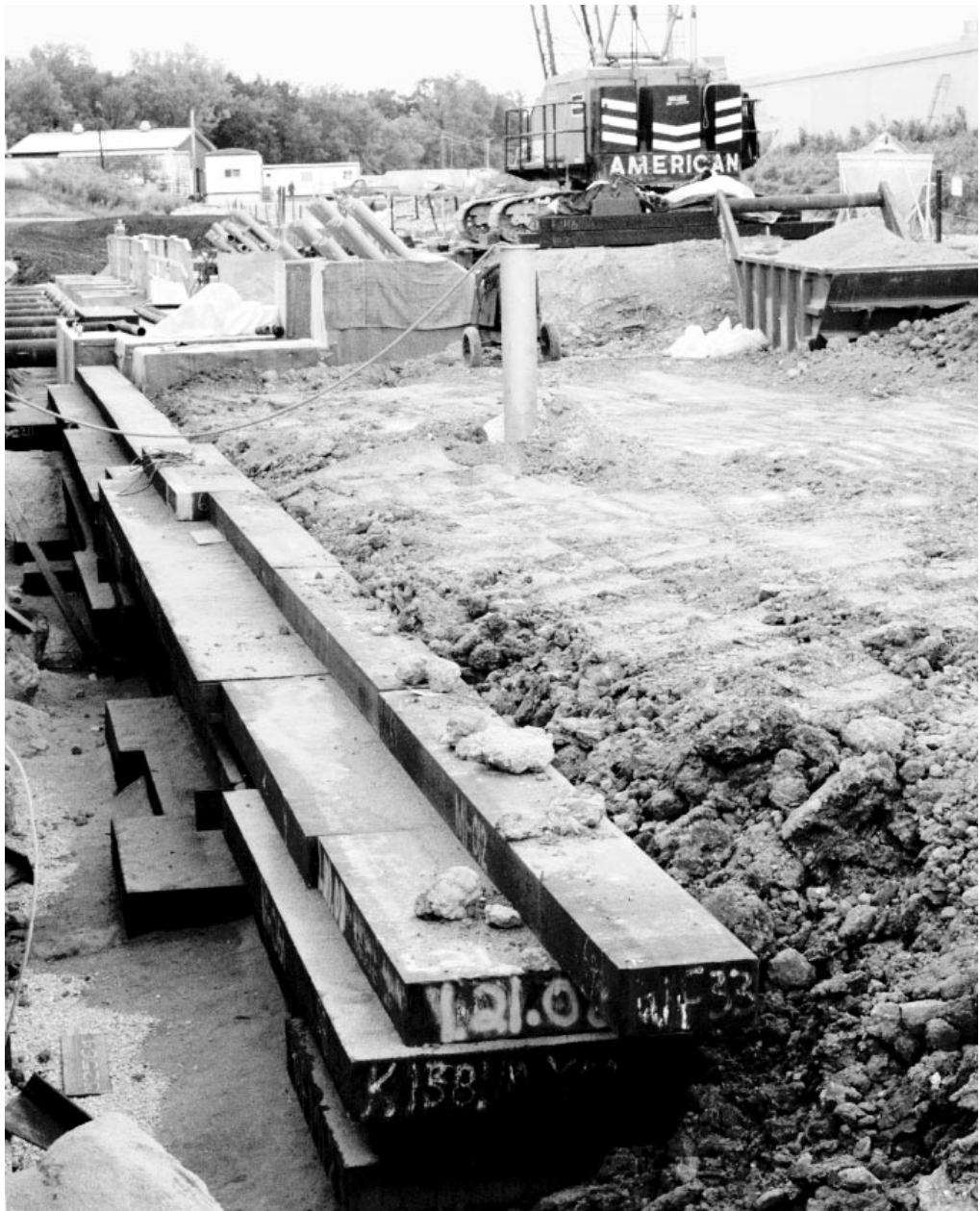
The reconfigured FZero tunnel segment uses about 4,000 tons of steel for radiation shielding. “If we put all 4,000 tons together, the steel would form a cube 25 feet on a side,” said Dixon Bogert.
