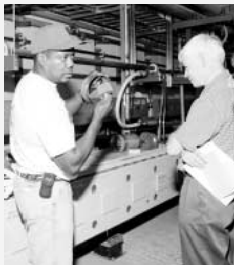
Paul Gentry demonstrates specially-designed tools used in the repair of the Low Conductivity Water (LCW) system.
