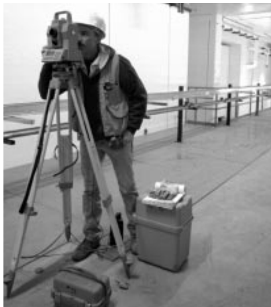
Gary Coppola surveys in the Tevatron tunnel.
