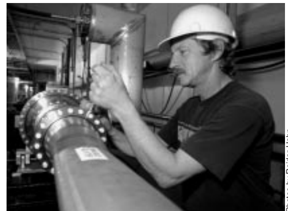
Keith Dillow works on installing the septum for slow spill extraction at the Main Injector.
