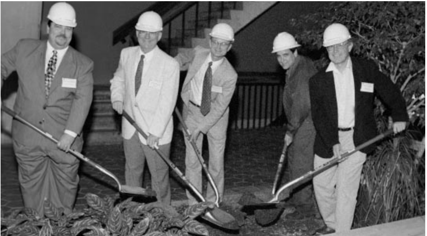
The official start of the NuMI construction: Robert San Martin, DOE (left), Dixon Bogert and Michael Witherell, Fermilab, David Ferguson, S.A. Healy Company, and Stanley Wojcicki, Stanford University, break ground in the planters of Wilson Hall.
