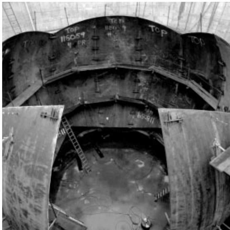
The construction of the 40-foot-diameter steel tank, from April to August, presented a major milestone. It will hold 250,000 gallons of mineral oil.
