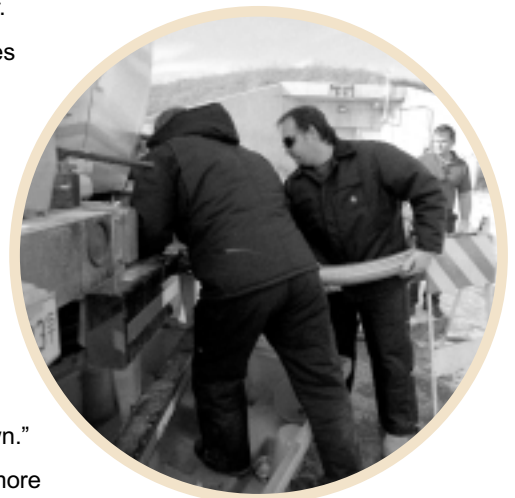
Fermilab technicians Craig Lerette (left) and Steve Sorenson pump oil from a tank truck into the MiniBooNE detector, located inside the building in the background. Lead technician Andy Lathrop (right) checks on the progress. It will take about 45 truckloads to fill the 250,000-gallon detector tank.
