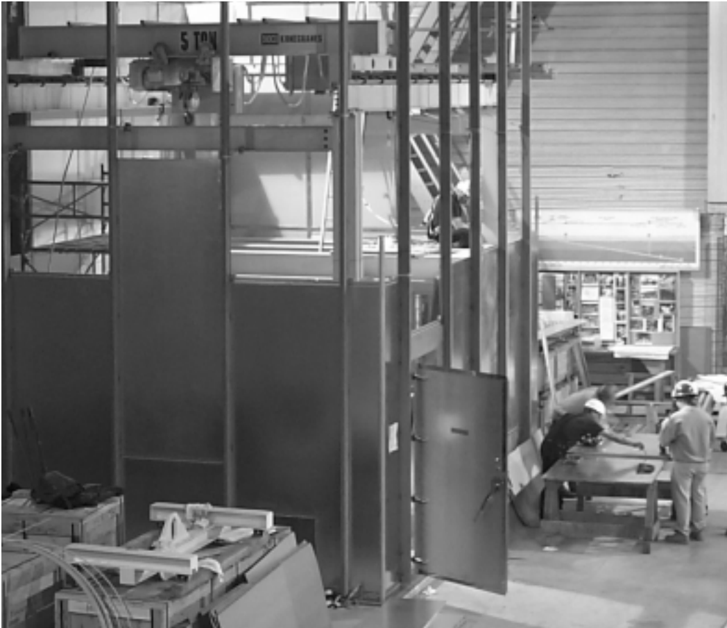
A clean room had to be built in the Soudan mine for assembling the cryostat. The completed facility (inset) houses an environment of only 10,000 particles per cubic meter. It is cleaned regularly with HEPA vacuum cleaners, and has a particle counter running continuously.
