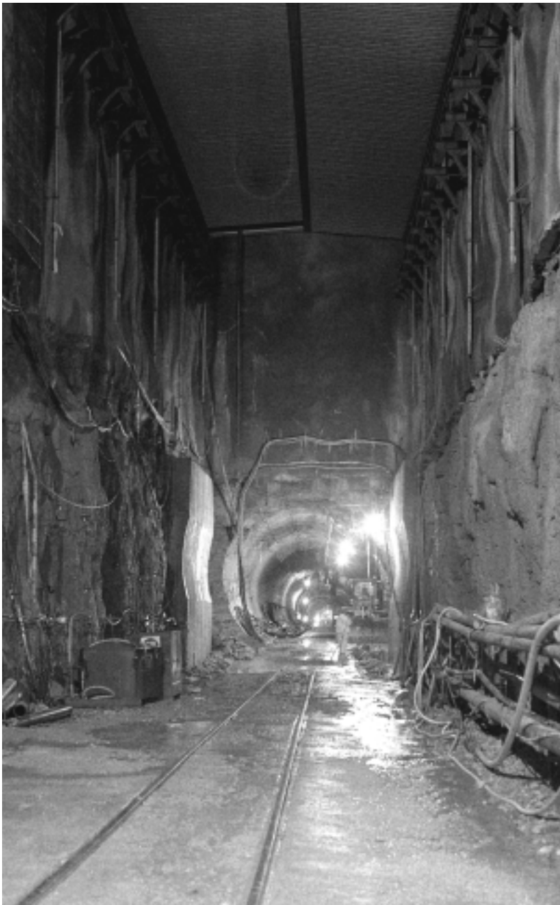
Miners completed the excavation of the NuMI target hall in January 2001. With a height of 60 feet and walls of rock, the hall's interior is reminiscent of a cathedral. The wall in the back shows the entrance to the decay tunnel.
